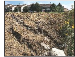
Soil erosion control
